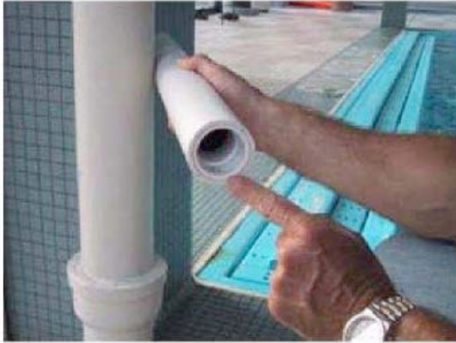
Sealed Retainer sleeve inserted into a two inch stock pipe
