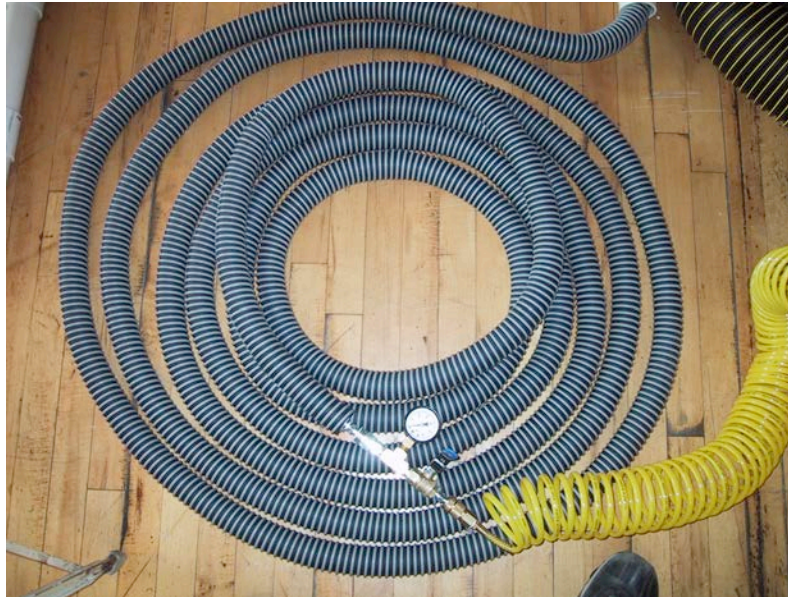
Pressure assembly connected to liner with shut-off valve in closed position
